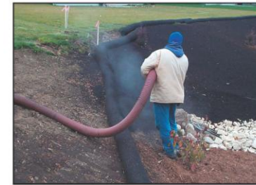
Pneumatic Installation of Media
