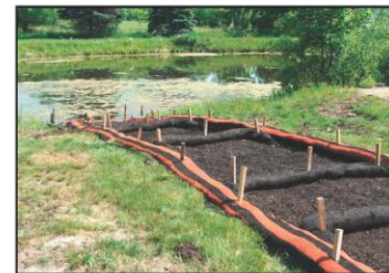
Installation of a Biofiltration System
