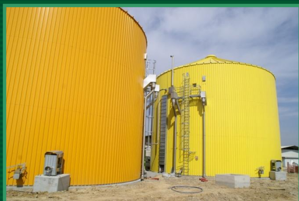
Vertical Anaerobic Digesters
