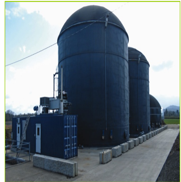
Lochmead Farms Digester
