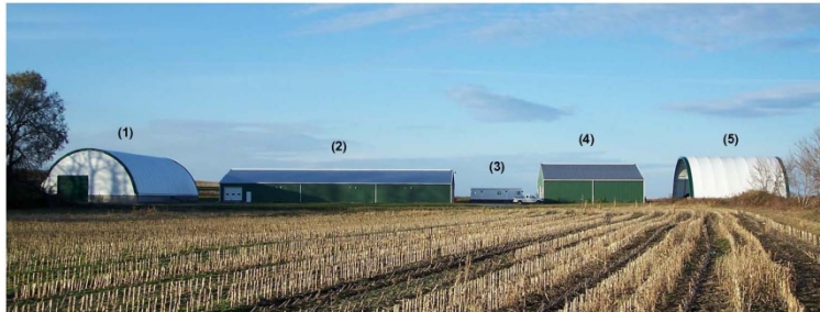
RT Solutions, LLC Vermicomposting Facility (Left to Right)
