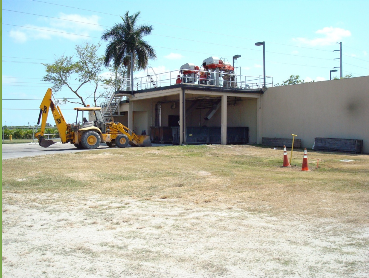
City of Homestead Waste Water Treatment Plant.
