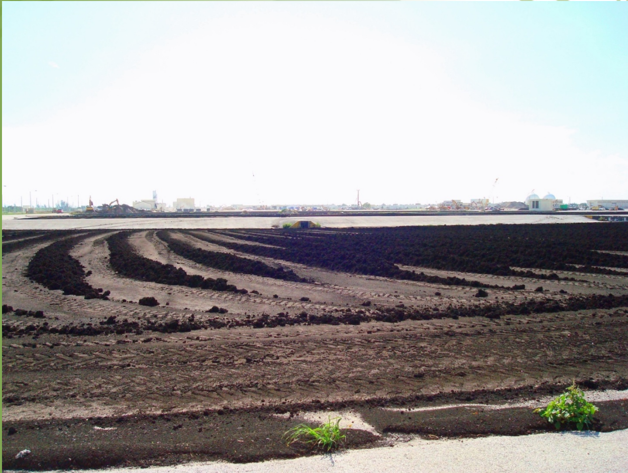
Solar drying beds at MDWSD South District Plant.
