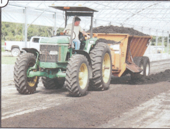
Blending wet bio-solids with dried solids provides inclement weather capacity
